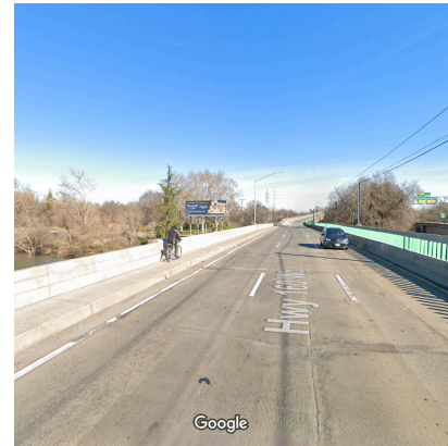
State Route 160 Bridge
